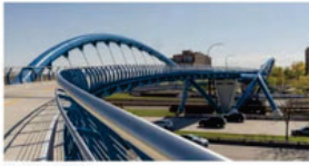
41st Street Bridge
